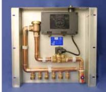
The Electronic Priming Assembly pictured is available in a single configuration but is capable of priming from thirteen to twenty separate floor drain traps from a single twenty one to thirty separate floor drain traps from a single control unit. The manifold is available in either 1/2" or control unit. The manifold is available in either 1/2" or 5/8" 5/8" compression fittings. This model serves 13 to 20 compression fittings. This model serves 21 to 30 drains.
