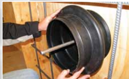
2. Attach Infinity® wall sleeve to locator cap.
