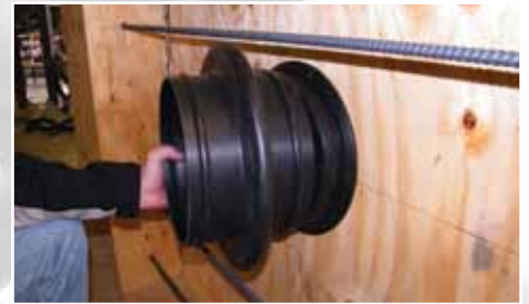
3. Cut the Infinity® wall sleeve \frac{3}{4} " shorter than the wall thickness (+/-1/4"), then insert the sleeve over the locator cap.
