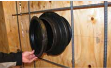
4. Insert the second locator cap.
