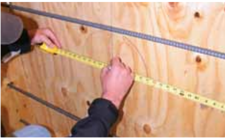
1. Using a tape measure, pull measurements from the horizontal and vertical positions to locate the center of the Infinity® wall sleeve.
