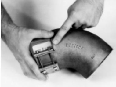
Step 1. Slide three-piece coupling assembly over end of piping to the positioning lug, or about one (1) inch on field cut pieces.
